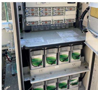
Macro cell site backup battery bank, Myers Flat, Humboldt County
